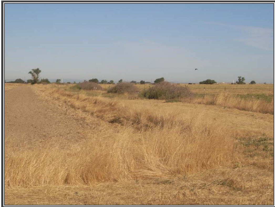
Photograph 3: Western edge of project site looking west. The berm running through the picture is on City-owned property and directs drainage from the project site into the ditch. Currently during large storm events, flows spill over the berm to the south, onto City-owned property.
